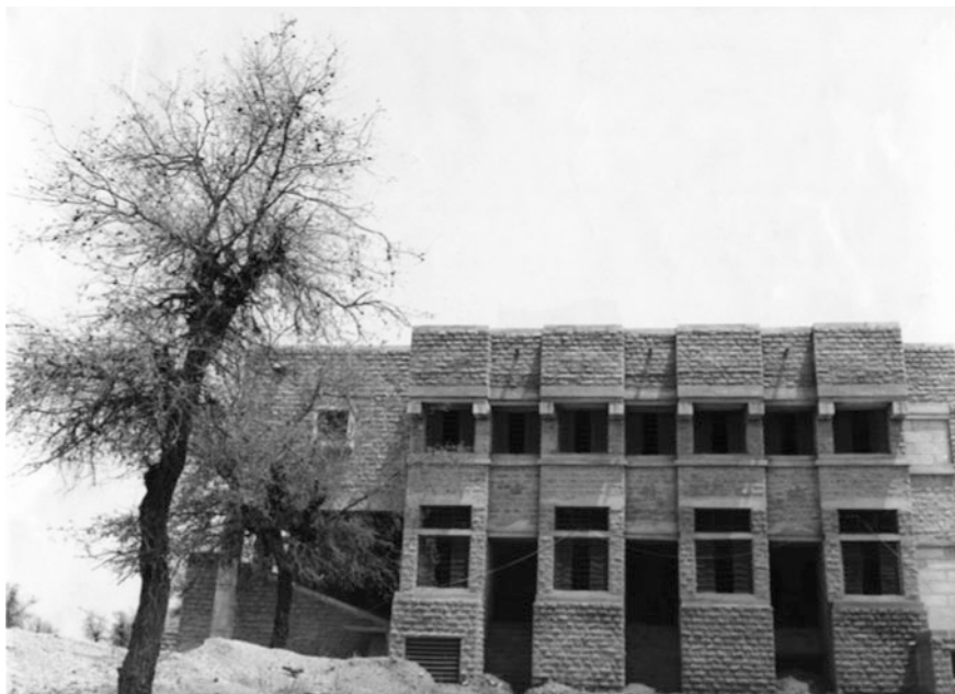
Fig. 4.15 Central library (courtesy architect Uttam C. Jain)
