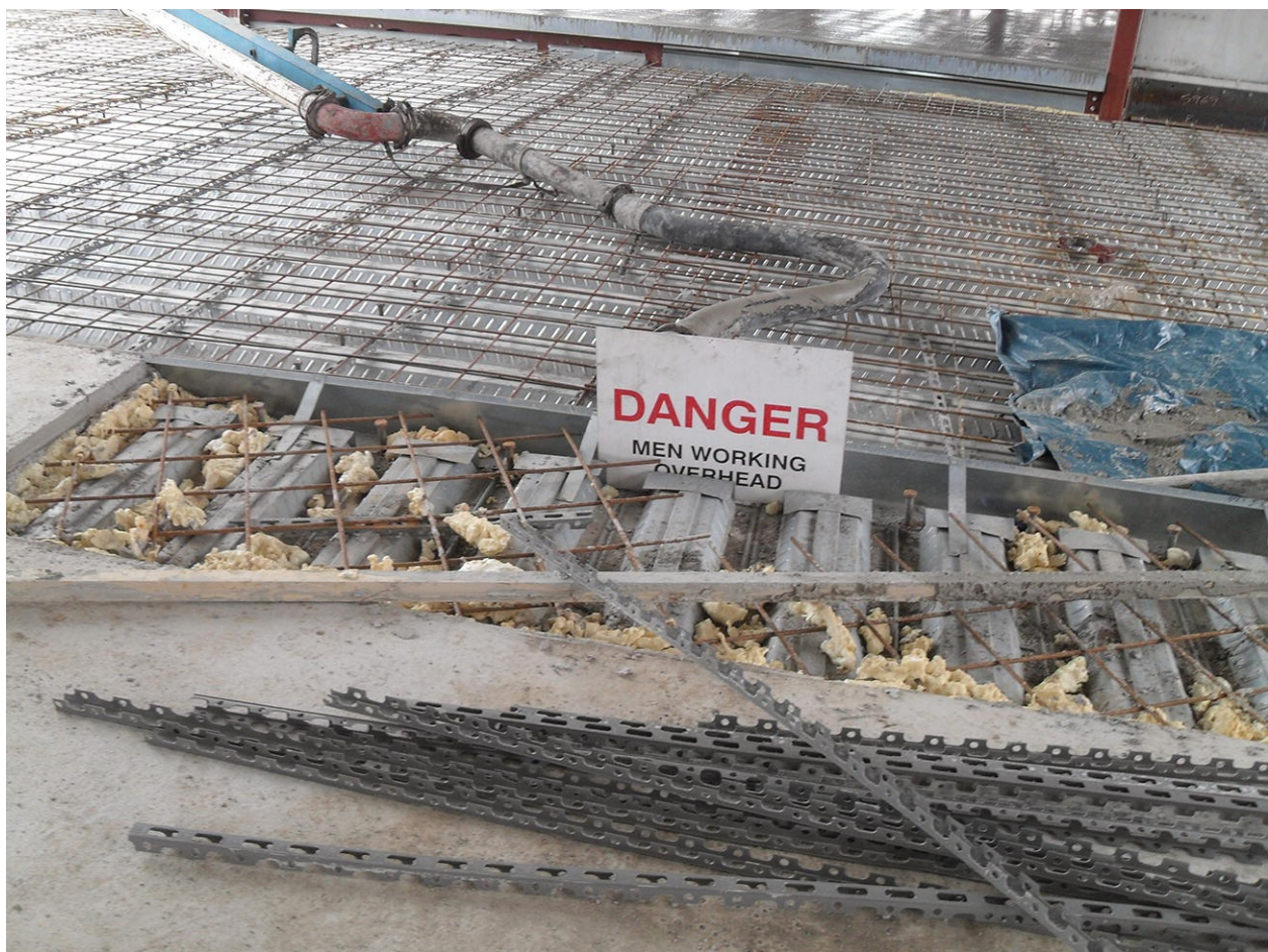
Figure 5.3 Danger – Men Working Overhead
