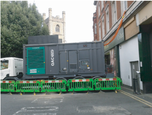
Figure 9.5 A generator providing a temporary electrical supply.
