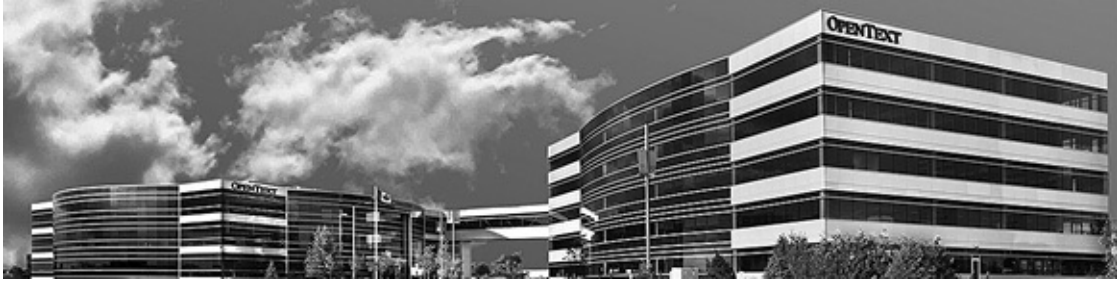
The OpenText headquarters.
