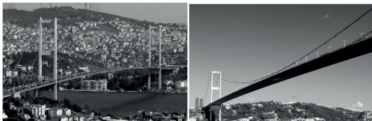
Figure 2. General views of the Bosphorus Bridge.
